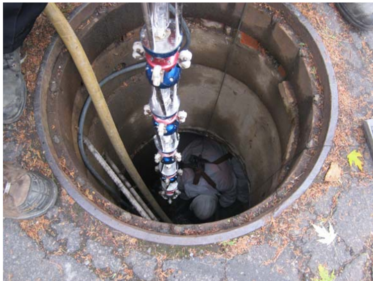
Figure 25 – Insertion du train de lumières UV
