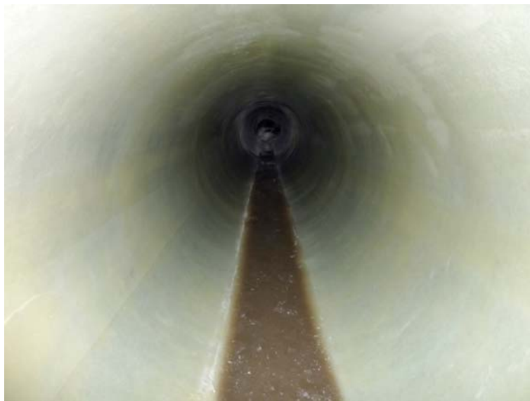
Figure 31 – Inspection de la gaine durcie (Source BKP Berolina)
