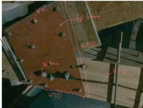
DÉTAIL RENFORCEMENT ET FIXATION DES CÂBLES AU NOEUD L0
