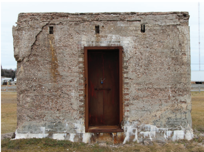
Figure 2 : Façade principale sud.
