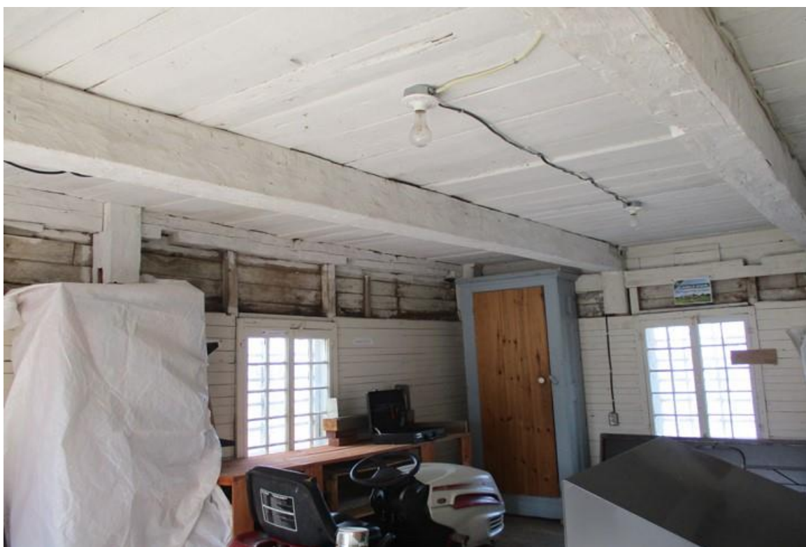
Photo 3: Structure existante supportant le grenier
