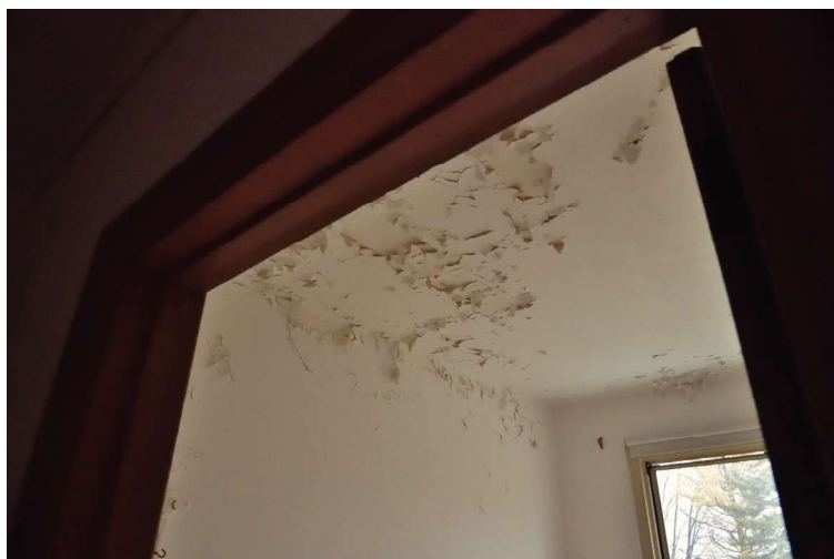
Figure 81. Infiltrations, BGLA
