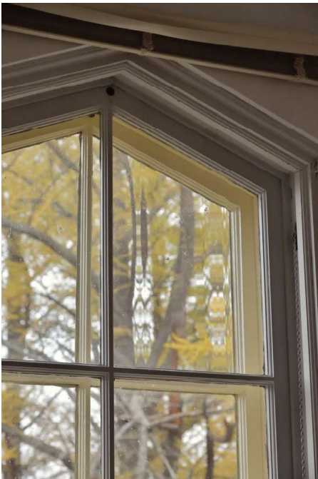
Figure 84. Fenestration originale, BGLA
