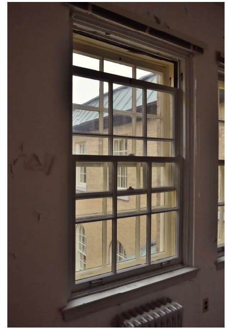
Figure 86. Fenestration originale, BGLA
