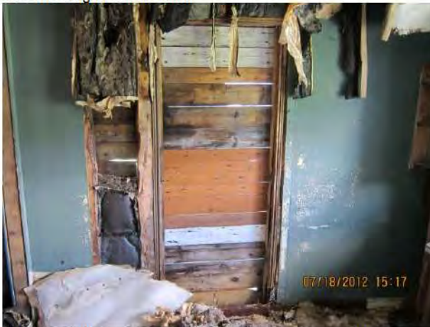
Image 26-HaGa-1, House: View of earlier door along west wall in work room.
