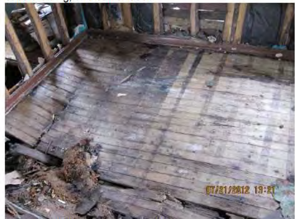
Image 24-HaGa-1, House: View of dining room floor and base molding.
