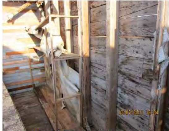
Image 12-HaGa-1, Shop: Shelving along east wall.
