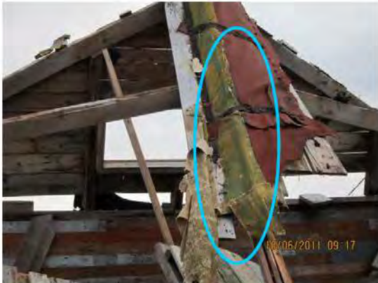
Image 1-HaGa-1, Shop: Roof apex with vapor barrier.
