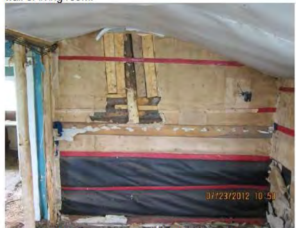
Image 35-HaGa-1, House: Structure of north wall, living room.
