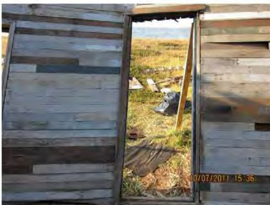
Image 3-HaGa-1, Shop: Inner covering of west wall.
