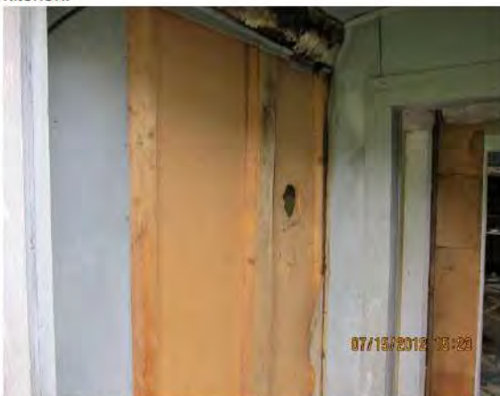
Image 33-HaGa-1, House: Structure of wall in north entrance.
