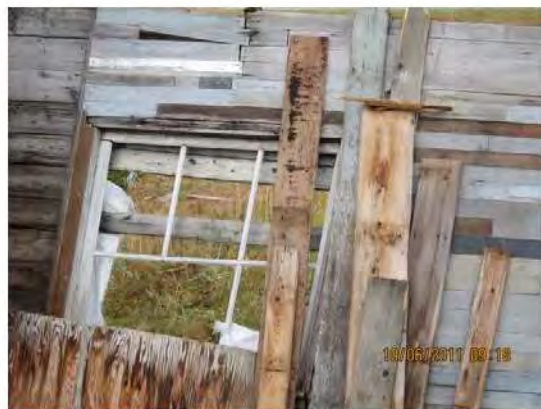
Image 5-HaGa-1, Shop: Remnants of west wall window.
