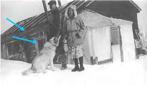
Figure 11a-Photograph depicting east wall of house taken around 1948 (Modified from Lofthouse 2012). Note: Presence of kitchen window and extension of roof.
