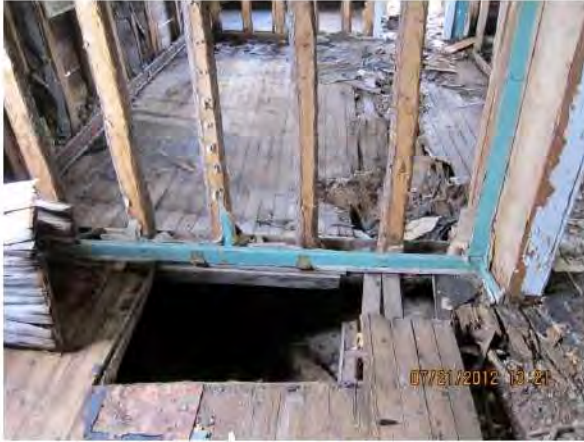
Image 25-HaGa-1, House: view of cellar entrance and floor molding in cellar room.
