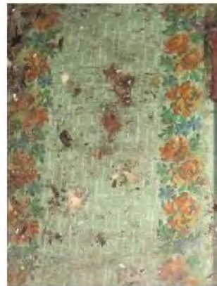
Image 47-HaGa-1, House: Floor covering along walls in living room, dining room, kitchen, hallway, and cellar room.
