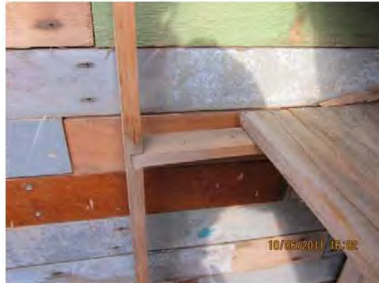
Image 4-HaGa-1, Shop: Inner covering of north wall.
