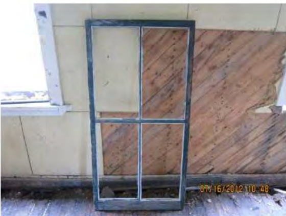
Image 15-HaGa-1, Church: Green painted surface of storm window (opposite side painted white).
