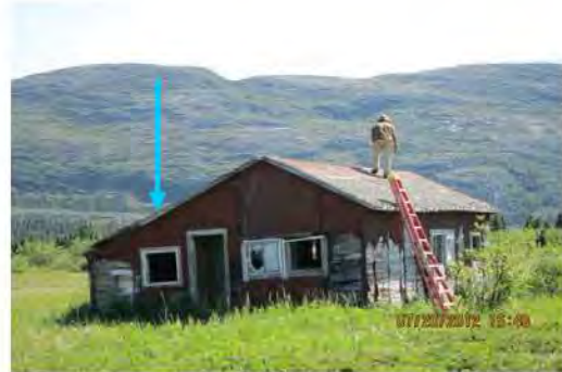
Figure 11b-Photograph of north side of the house taken during the 2012 field season. Note: Change in roof angle.
