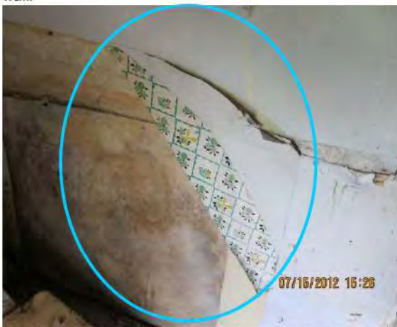
Image 32-HaGa-1, House: Earlier wall covering in kitchen.
