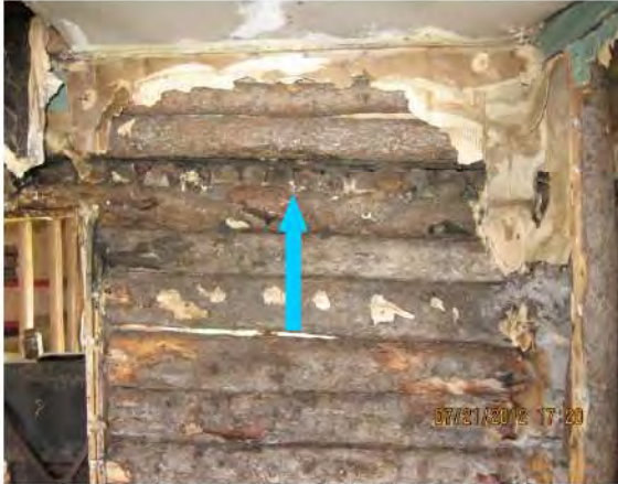
Image 31-HaGa-1, House: Cellar room view of east wall.
