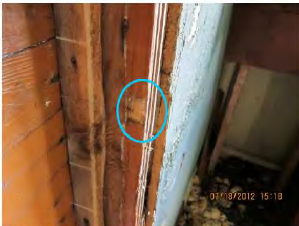
Image 27-HaGa-1, House: Hinge/latch mark on frame of earlier door in work room.
