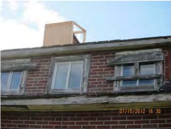
Image 14-HaGa-1, Church: Outside view of 2 nd floor windows along east wall.
