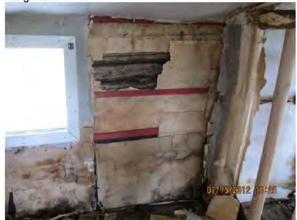
Image 36-HaGa-1, House: Structure of east wall, living room.
