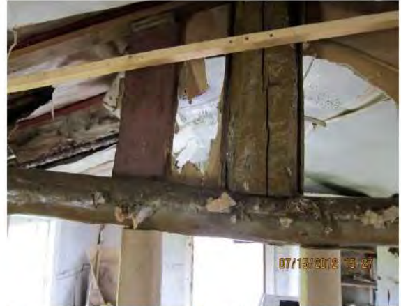
Image 34-HaGa-1, House: View of chevron (?), south wall of living room.
