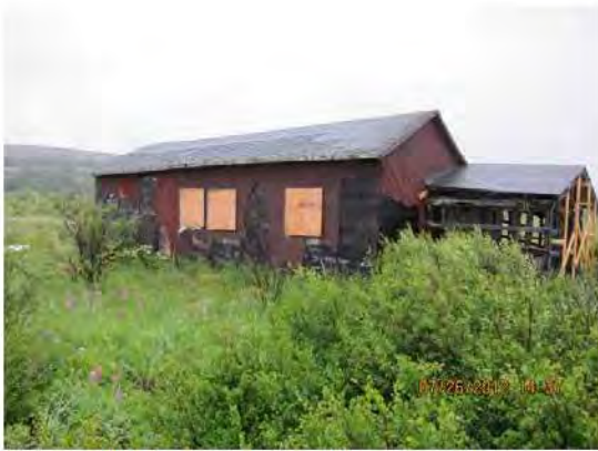
Image 43-HaGa-1, House: Outside view of west wall.
