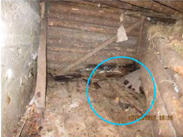
Image 37-HaGa-1, House: North view of cellar. Note remains of shelf structure.
