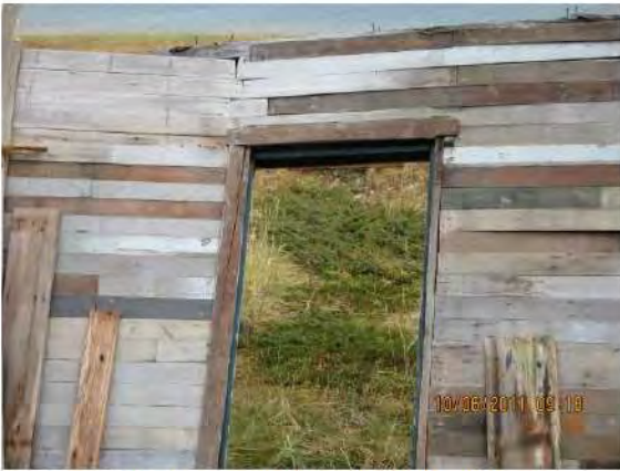
Image 7-HaGa-1, Shop: Inside view of door frame.
