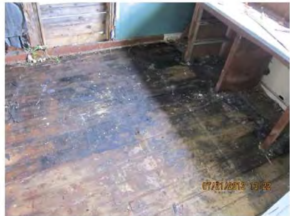
Image 23-HaGa-1, House: View of workroom floor, base molding, and earlier door.
