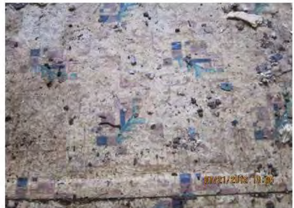
Image 46-HaGa-1, House: Floor covering in work room.
