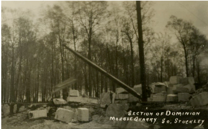
Figure 6.22 Dominion Marble Quarry, Stukely-Sud S.A. [1911?], BAnQ Rosemont-La Petite-Patrie, CP 029146 CON
