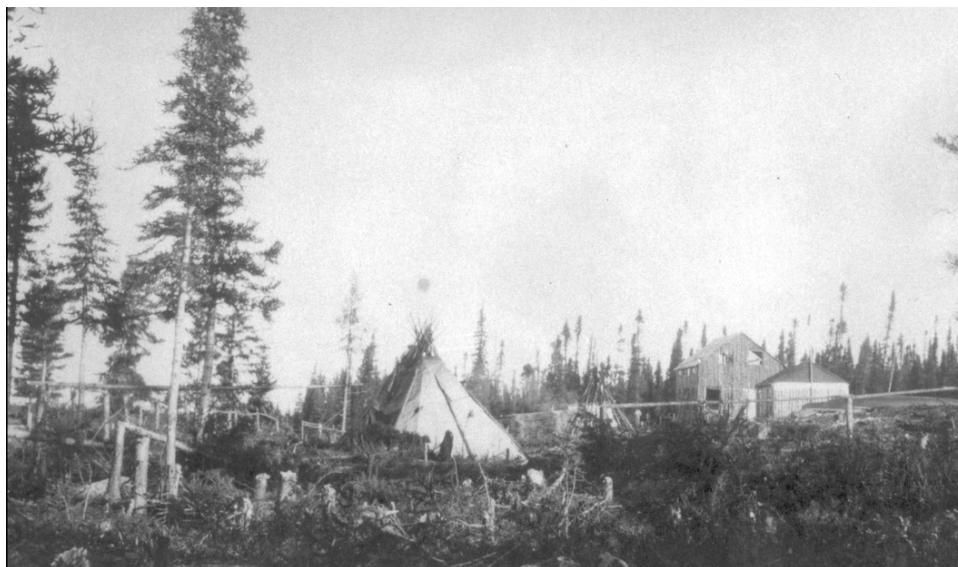
Figure 5.16: Fort McKenzie outpost under construction in 1917 showing Naskapi tipi, or iyyuuchiwaahpuch , and tipi frame (foreground). Photo by Olhaus Murie. From Hammond ( in progress : fig. 2-17).
