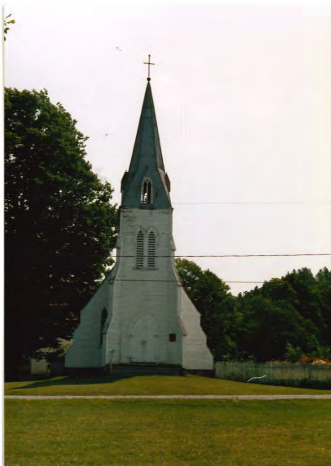
Ways Mills. Church of the Epiphany. La façade.
