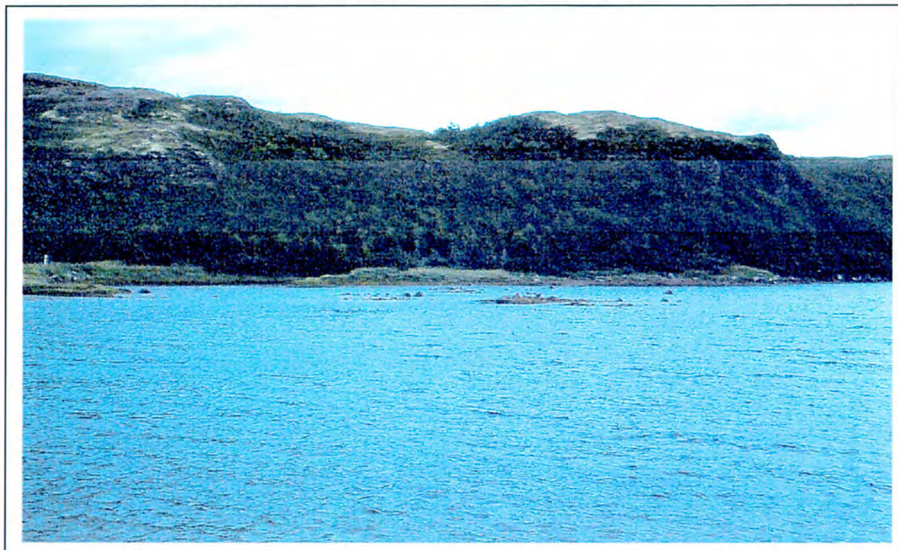
Figure 13 Eastern part of Baie du Vieux Fort: Zone C, looking southeast (Film I, No. 28).
