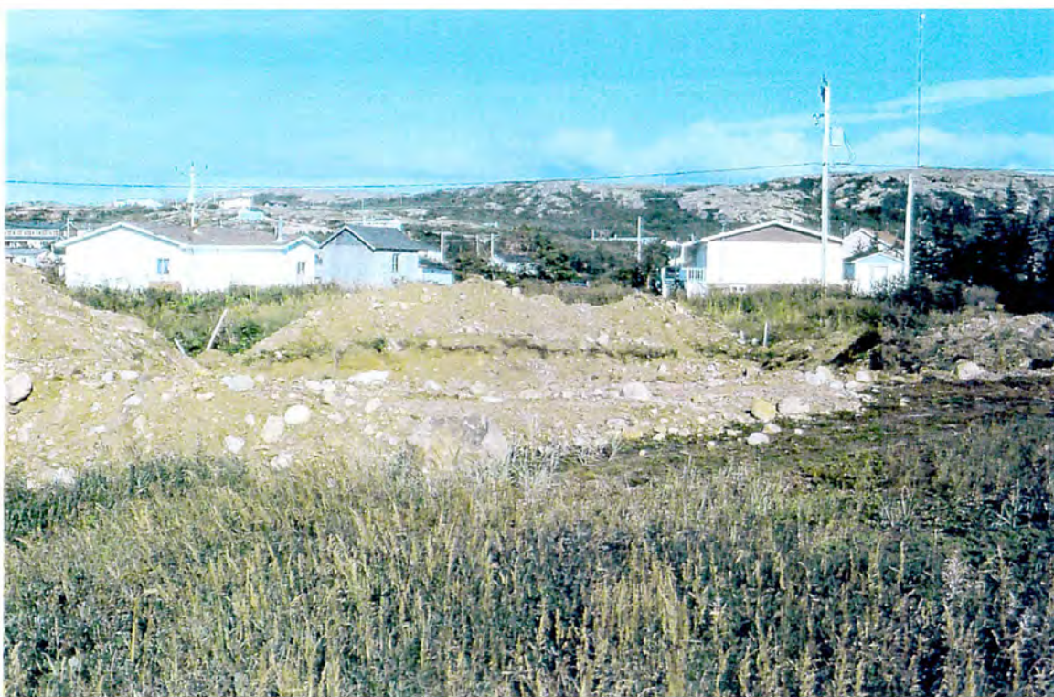
Figure 24 Eibk-49: excavation for the house to be moved to the point, looking west (Film 2, No. 9).
