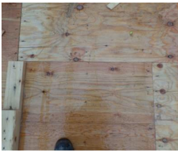
Photo 1 - clouage conforme
