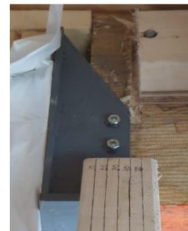
Photo 8 - appui insuffisant
