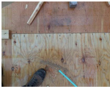
Photo 2 - clouage conforme
