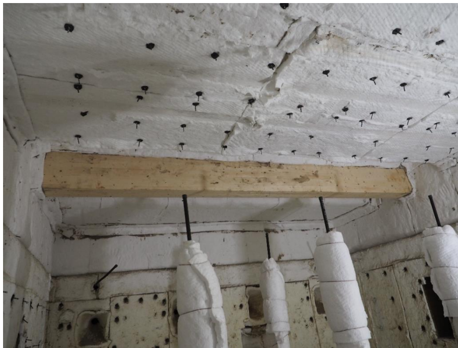
Figure 4: The Beam inside the furnace
