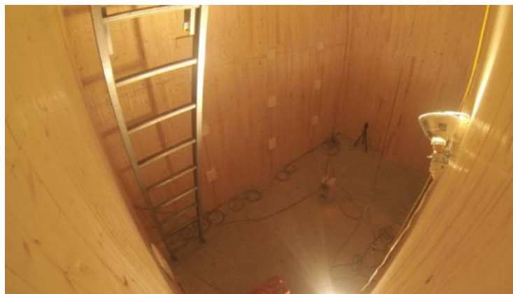
Figure 13. Instrumentation inside the stair/elevator shaft.
