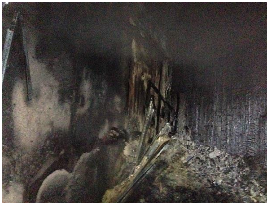
c) Interior of the fire room
