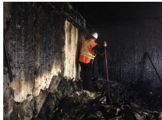
d) View of the shaft wall from the fire room
