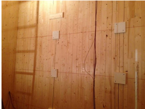
a) Interior wall of the shaft
