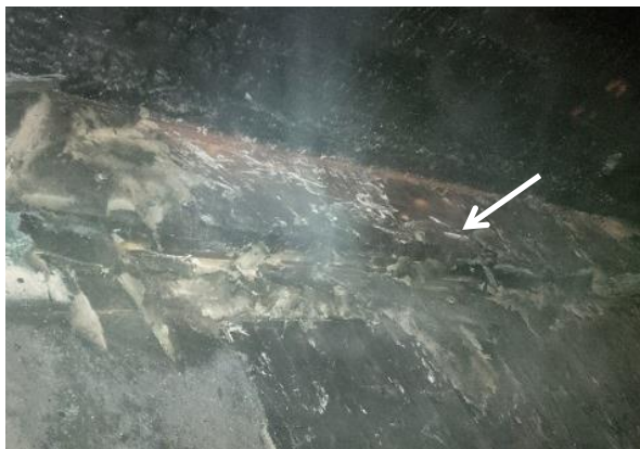
e) Ledger beam in place and lightly charred
