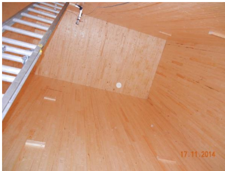
Figure 8. Interior of the stair/elevator shaft.
