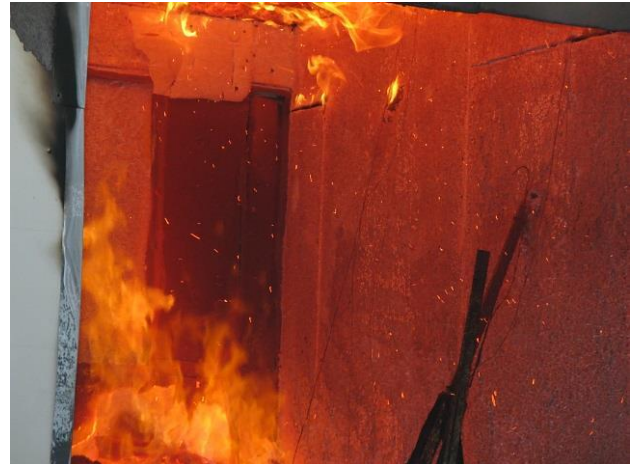
d) &gt;1.5 h, some insulation and gypsum still in place
